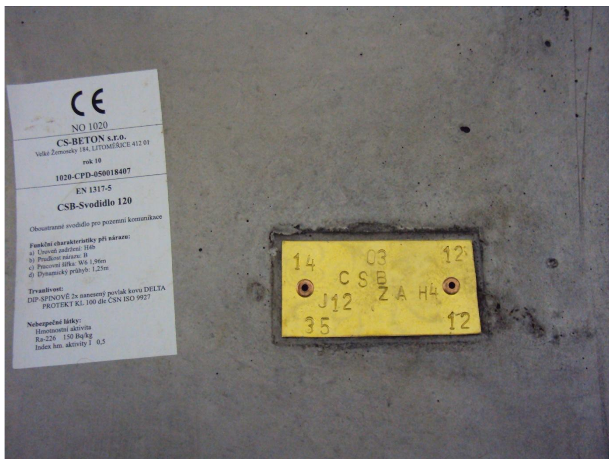
Figure 12 – CE label and brass label marking CS BETON concrete barriers
