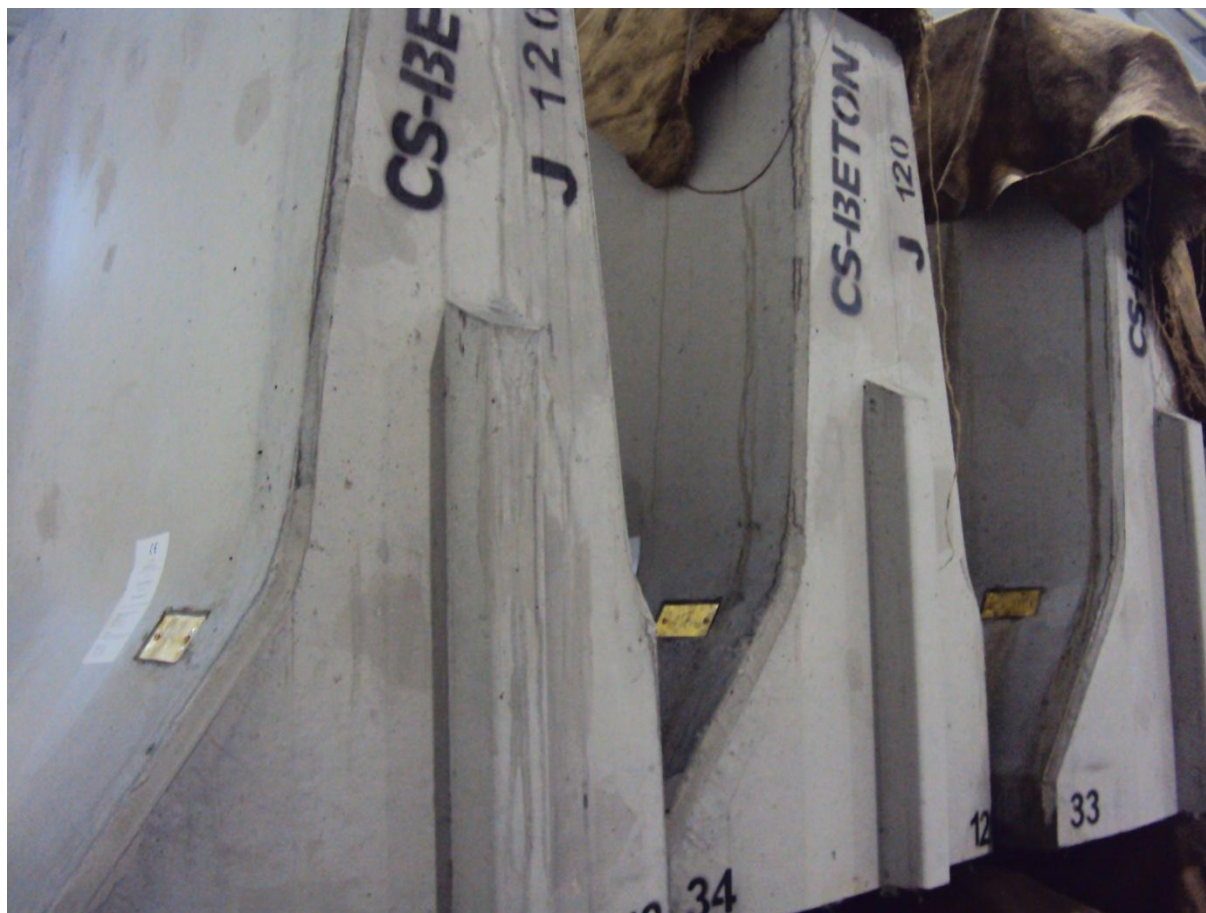
Figure 15 – Colour coding at one end of each section
